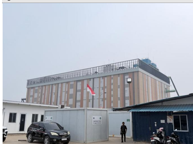
Figure 1. NeutraDC BTM-1 data center
