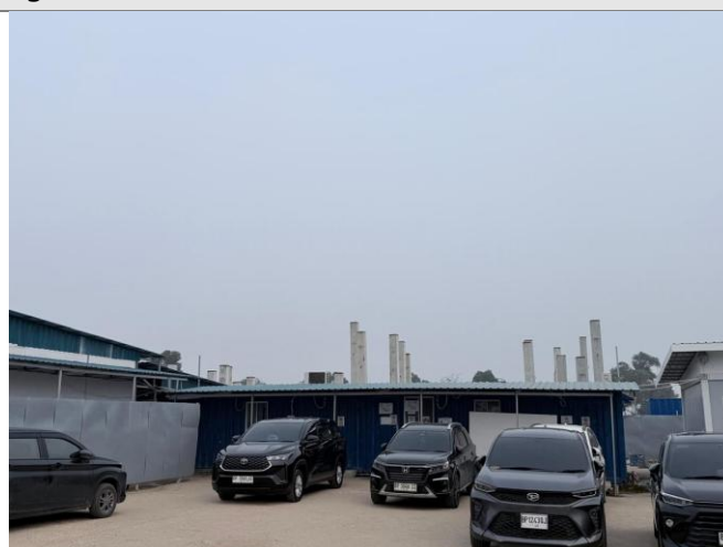
Figure 2. NeutraDC BTM-2 data center under construction
