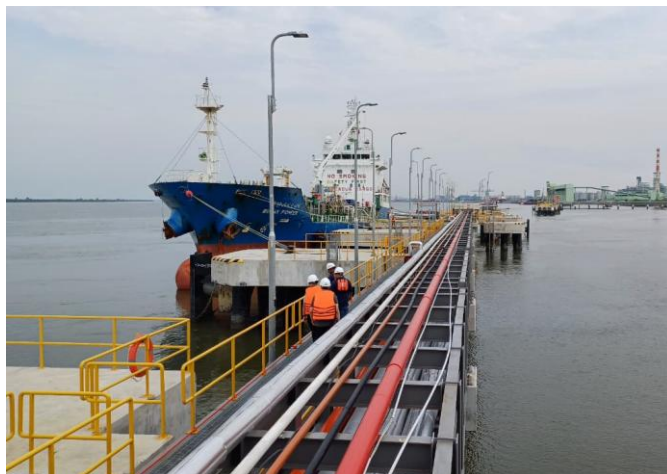
Figure 28. STAOF dedicated jetty port
